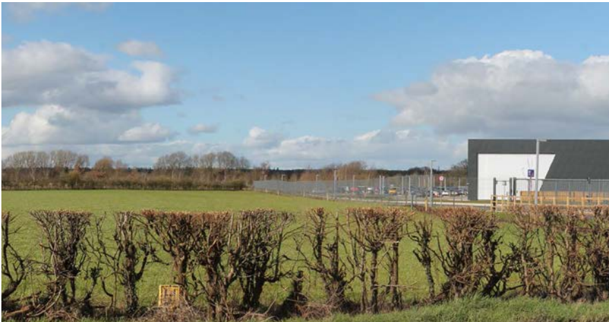
Figure 8: Southern boundary of the site facing north
